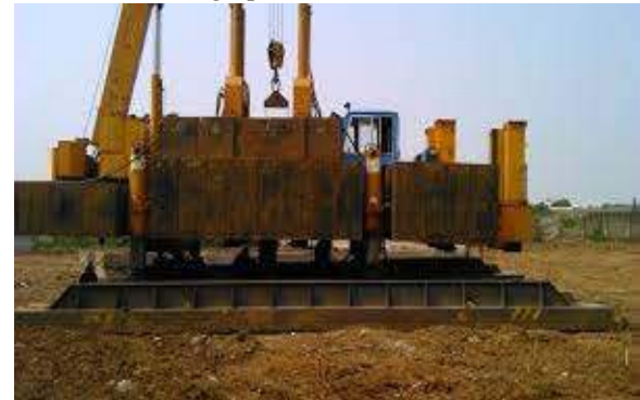
Gambar 3. 2 Hydraulic Static Pile Driving
