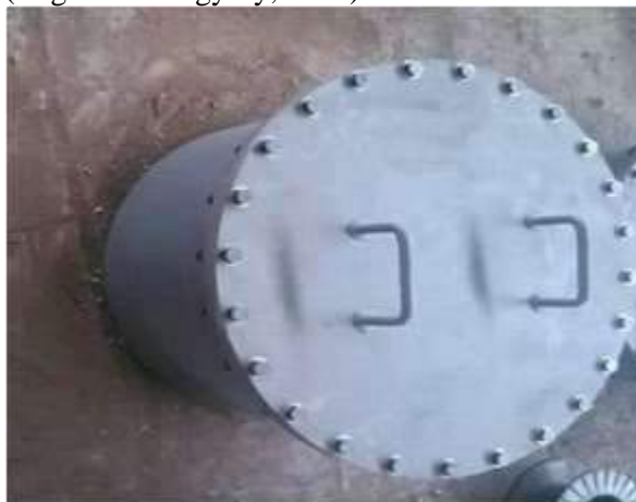
Gambar 6. Man hole (Lobang lalu orang) diameter 10 inc.
